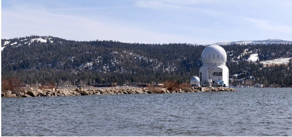
Figure 1. Big Bear Solar Observatory with the new 5/8-sphere dome. The small dome in front of the observatory building houses an auxiliary telescope for Earthshine observations.
